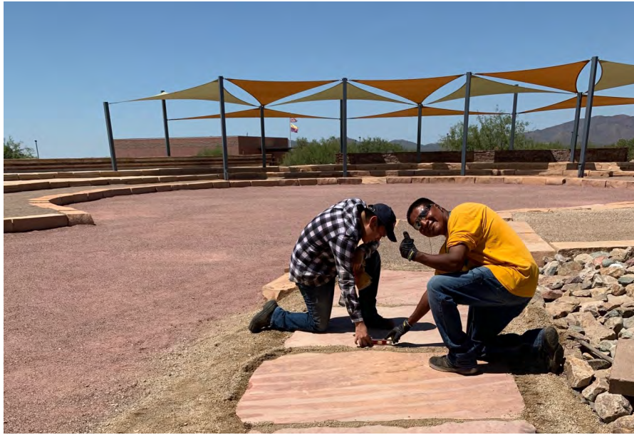
Carpentry Apprentices Kade Claw and Angel Moreno measure the slope of the flagstone ramp leading to the amphitheater. The ramp meets the Americans with Disabilities Act standards of accessible design. Photo by Robert Wambolt.
