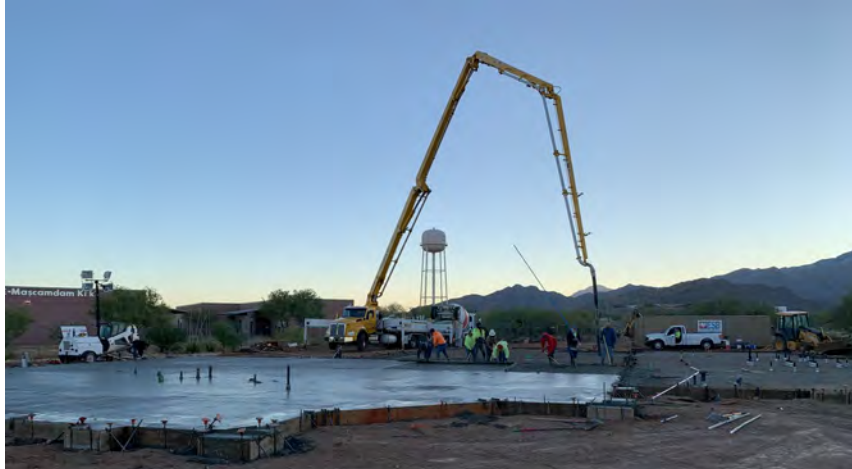
The foundation slab was laid in November 2020. Photo by Robert Wambolt.
